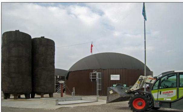
On top of the post-digester, there is a gas storage mounted. From there, the raw gas is fed to the CHP-units. All substrata are mixed up in a 200 m<sup>3</sup> premixing pit. From there, the substrata can be pumped directly into the digesters. Two tanks with fat and glycerin stand on top of the premixing pit. They are heated and insulated in order to keep the material liquid which is pumped directly into the digesters.
