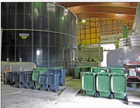
Food waste is arriving in bins. They are emptied into the sanitizing unit which chops, stirs and heats up the material.
